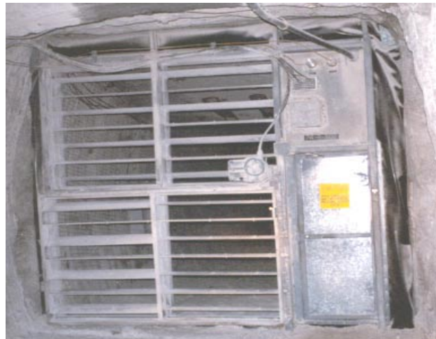
FIG. 22 - An example of a louvre regulator.
